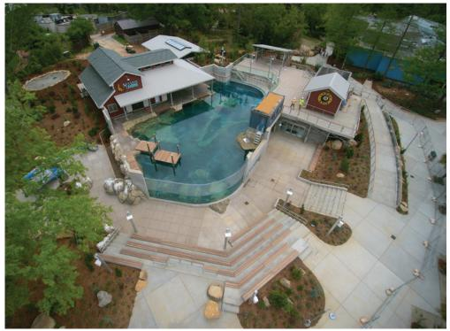
The Life Support Systems treat 250,000 gallons of water, turning over the complete volume in one hour. Water is monitored and measured for temperature, salinity, oxygen and bacteria, etc.
