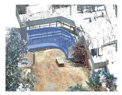
ensuring the fabricator was provided with exact dimensions to create the curved acrylic panel, with any adjustments verified and approved by designers – resulting in a perfect fit for installation when the materials were received on site.
