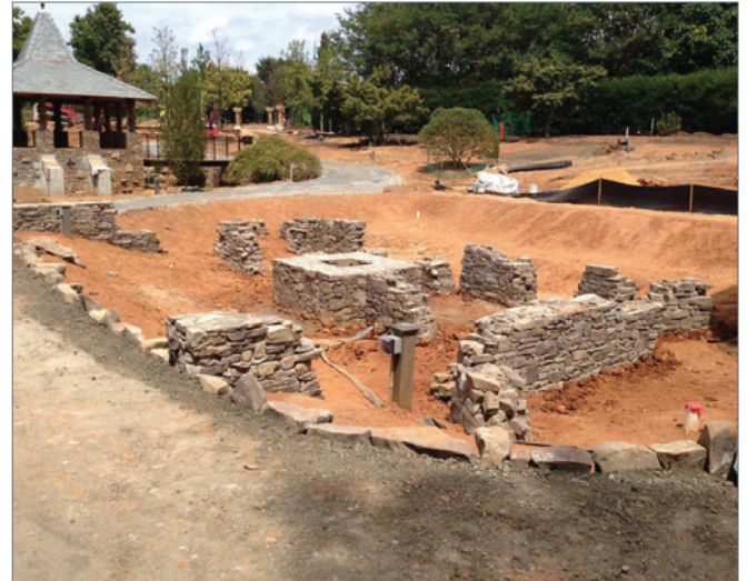
• Sunken Pond in progress
