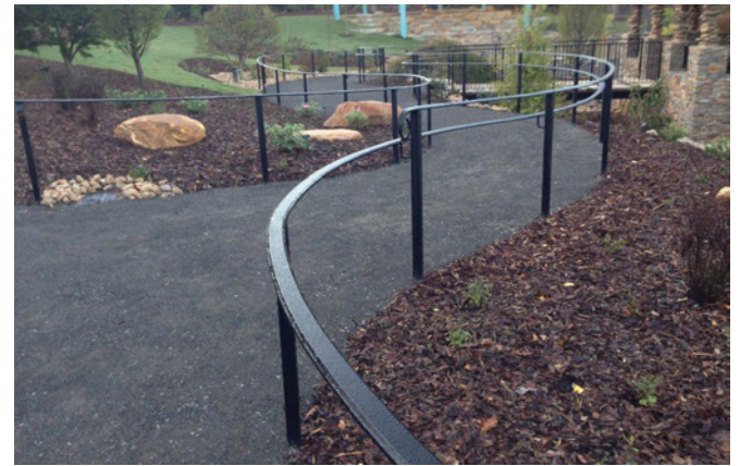
• Milled asphalt pathways featuring custom handrails created by forging bar stock steel along the curves
